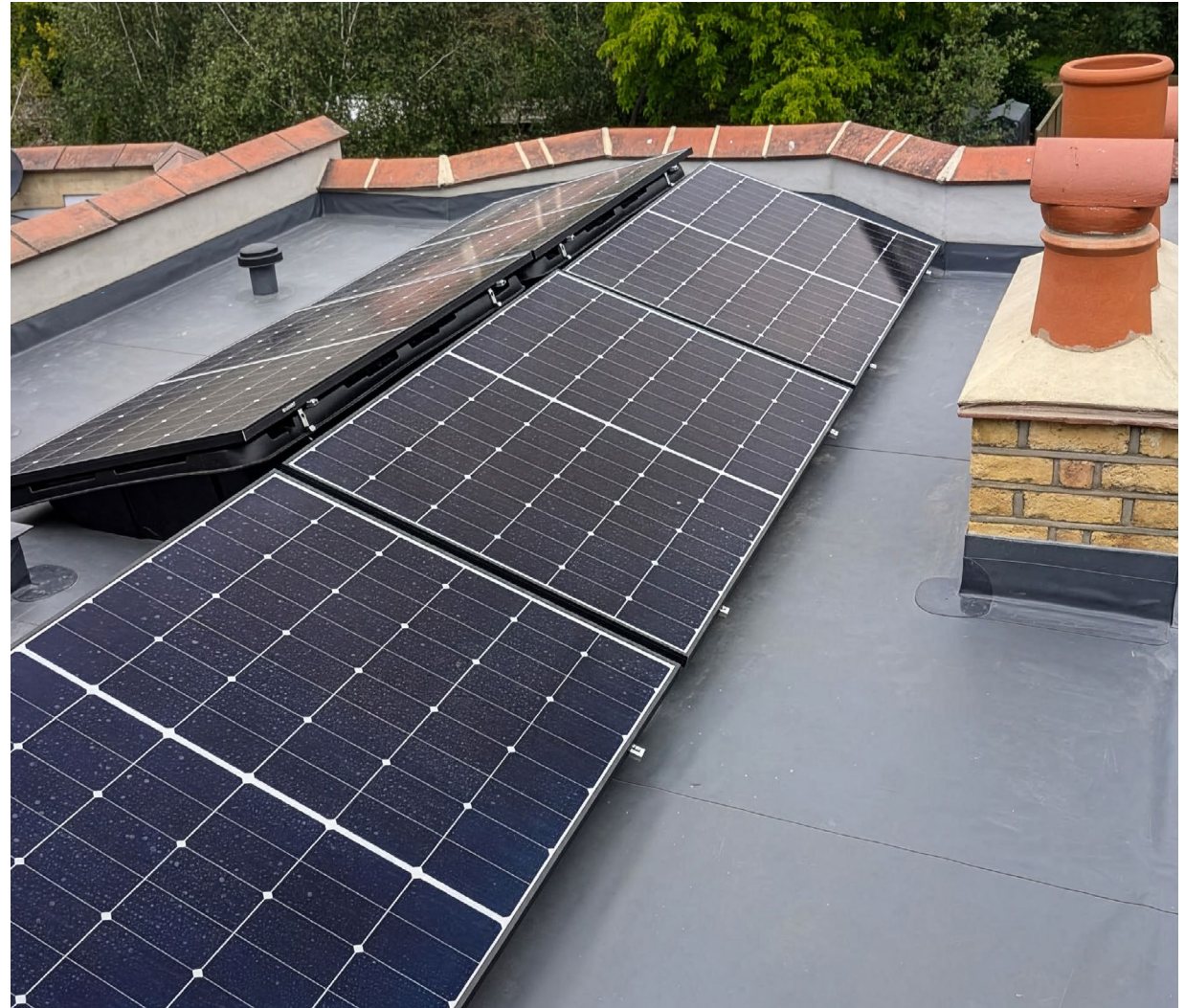
Photovoltaic solar panels on the flat roof of the rear addition. New rooflights were triple glazed.
