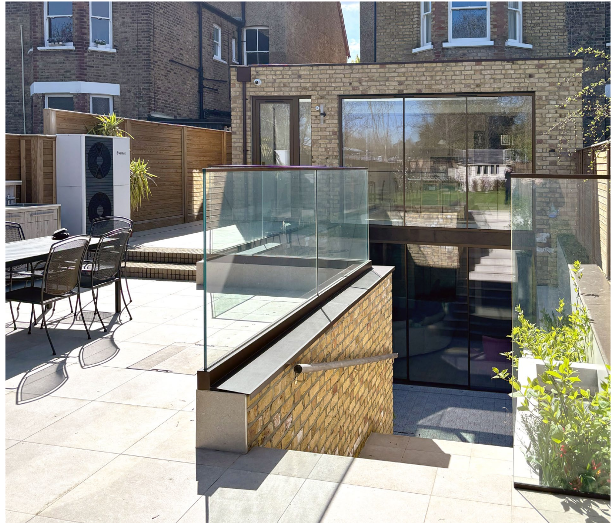
The rear single storey extension and lightwell to the new basement.
