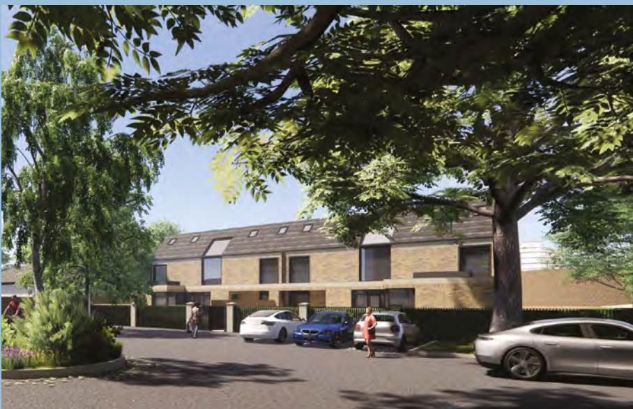
Work to build two Passive Houses commenced
