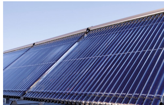
A Solar Thermal Collector is made up of glass tubes with a vacuum to capture the sun's heat and transfer it to provide hot water.
