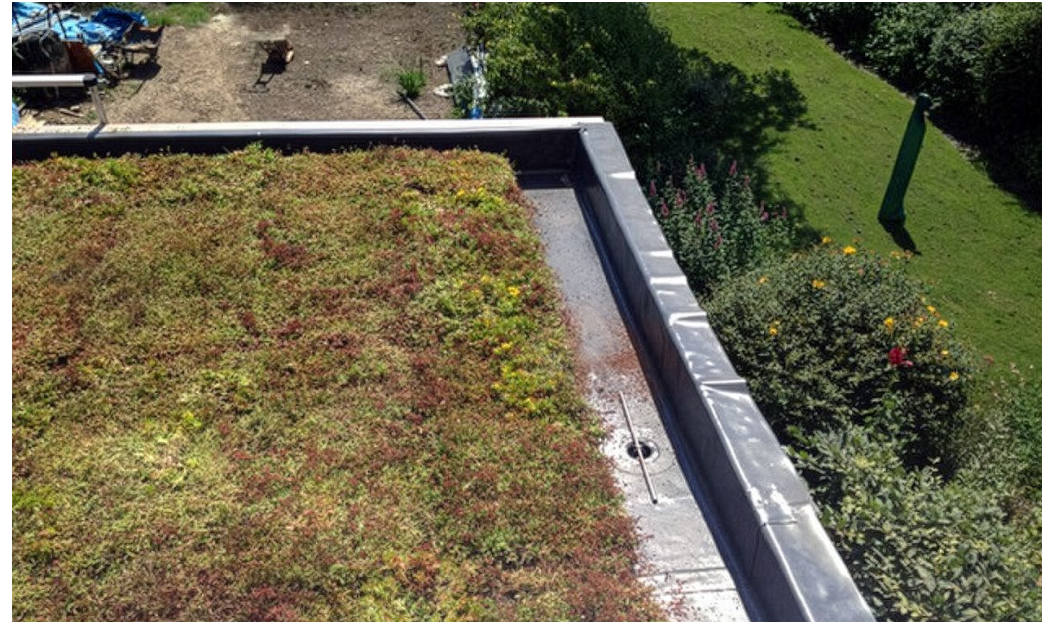
The extension roof was designed to be planted with sedum, which reduces rainwater run-off, supports insects and looks much more interesting than a bare roof.
