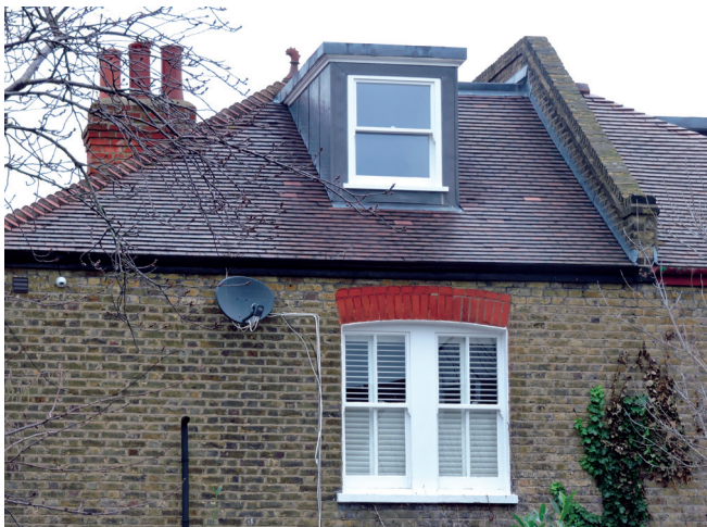
Visually unobtrusive satellite dish
