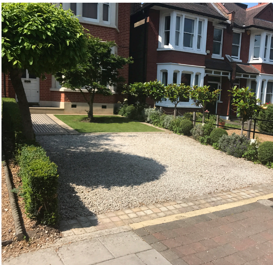
New hardstandings should incorporate permeable materials and attractive landscaping to help retain a green and biodiverse streetscape
