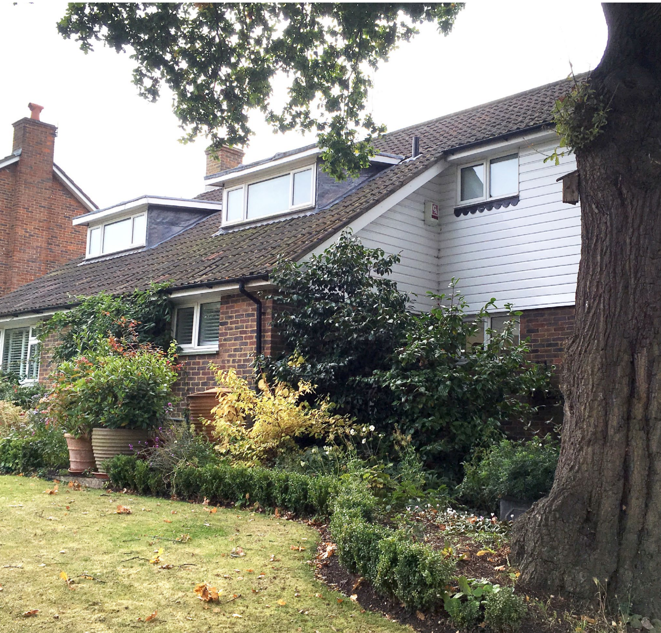
Before the works commenced. The new side extension is not visible from the street
