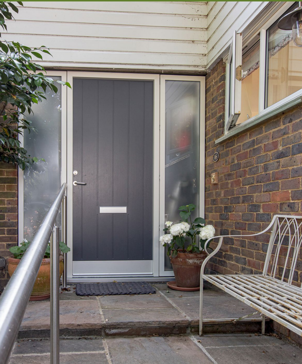
The front door and windows have been replaced with thermally efficient products
