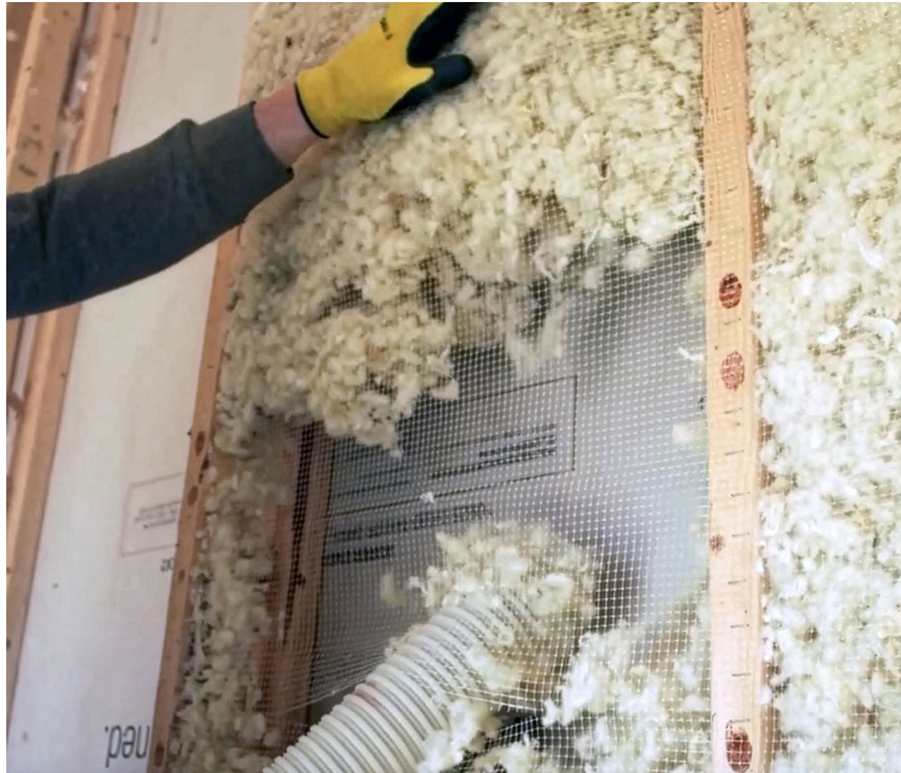
Blown wood fibre insulation being installed
