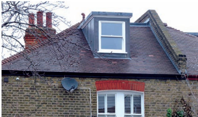
Visually unobtrusive satellite dish
